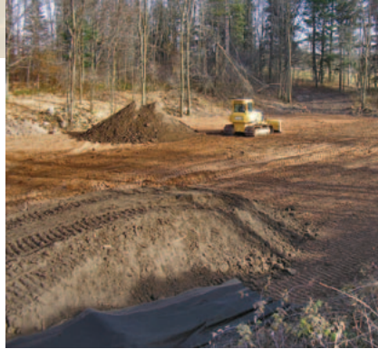
Runoff from 300 acres flowed into this large sinkhole and drained to groundwater. The sinkhole was capped with soil, and a pipe was installed to divert the runoff.
