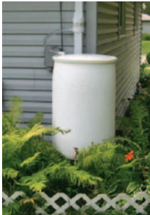
A rain barrel is a low-cost way to reduce runoff from the roof.
