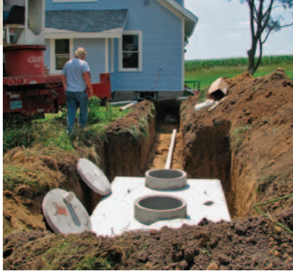
A new septic system replaces one that was malfunctioning.
