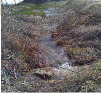
Report observations of water suddenly disappearing in a road ditch to the township or county road department. This may indicate a new sinkhole.
