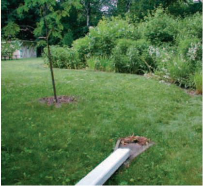
A downspout and swale control the direction of roof runoff.
