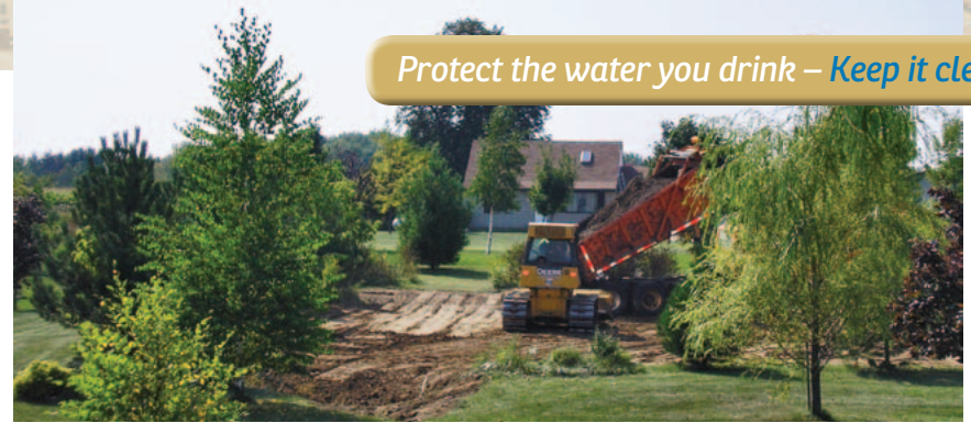
Yards may need to be re-worked to divert runoff from sinkholes, fractures or old wells. Here a man-made pond collected polluted runoff from the surrounding fields, yard and road ditch, but never held water for long. It drained through a bedrock fracture, repeatedly contaminating groundwater. The pond had to be filled-in and the yard graded to stop the contamination.
